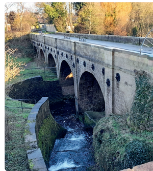
Viaduct at King's Mill Reservoir
