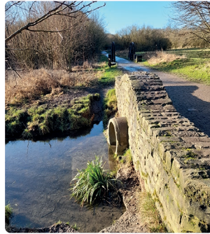
Bridge over the river
